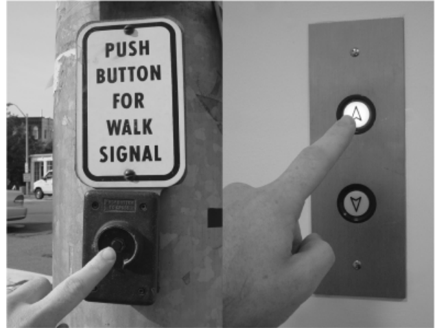
Figure 6. “Walk” Buttons Do Not Acknowledge Actions Like Elevator Buttons Do
